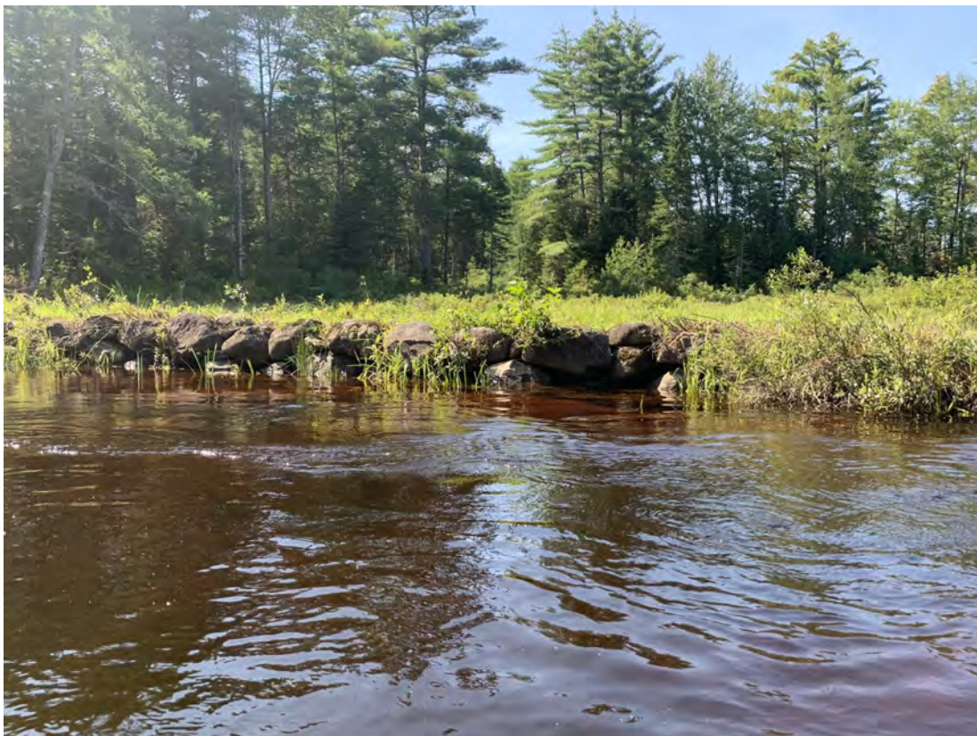
Photograph 22: Revetment at downstream end of Melvin 3
