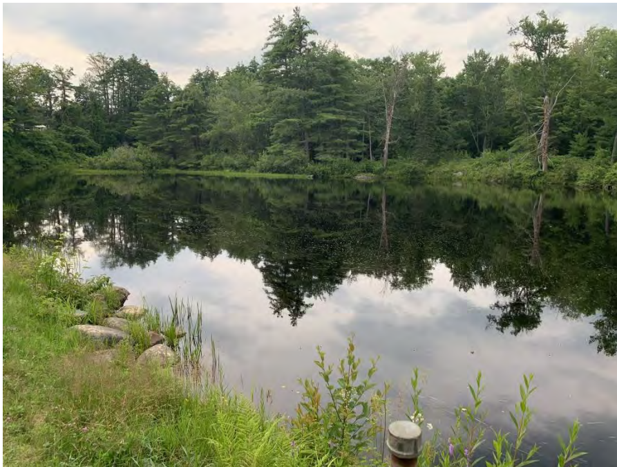
Photo 6. The Pope Dam impounds and widens the Melvin River's channel.
