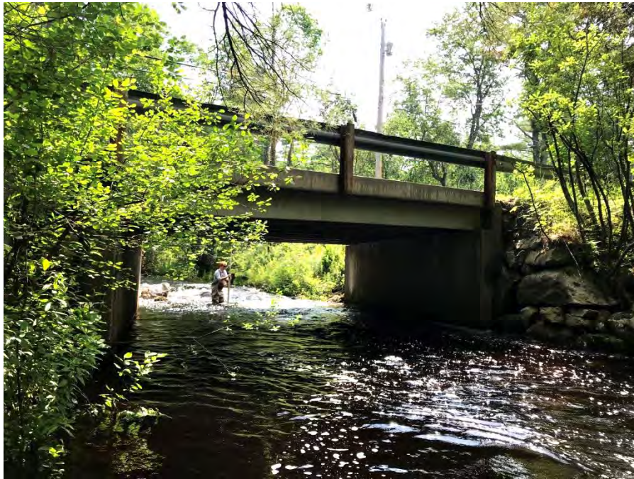
Photo 41. An open-bottom bridge conveys flow of Reach 5 under Sodom Road.
