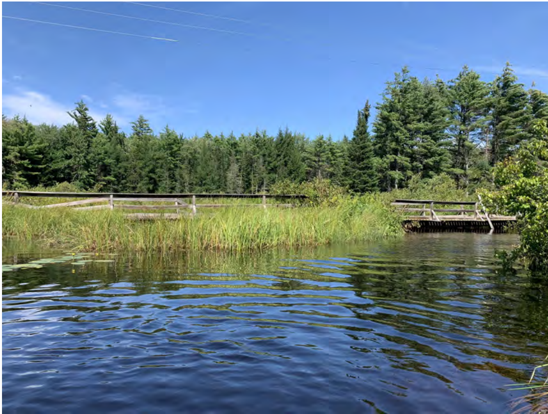
Photograph 21: Snowmobile crossing at downstream end of Melvin 3
