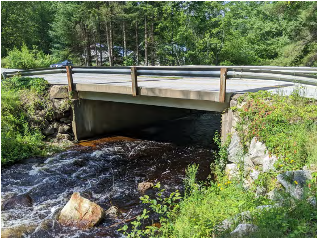
Photograph 16: Sodom Road crossing of Melvin River
