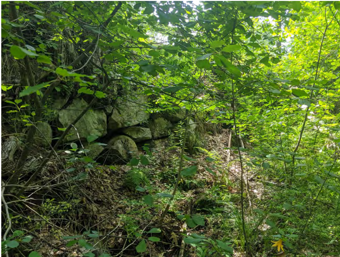
Photograph 17: Masonry on downstream slope of Sodom Road, potentially former dam
