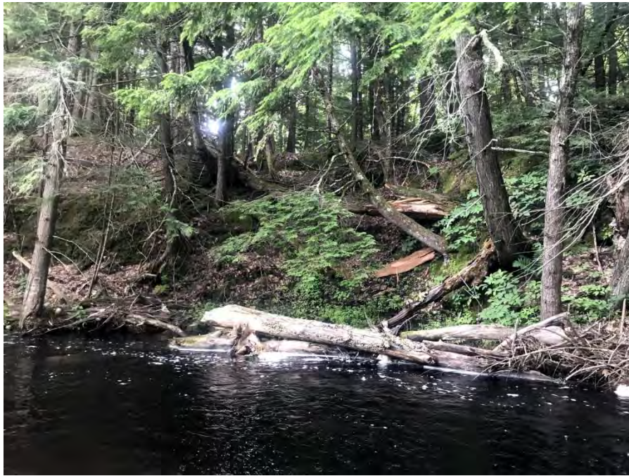
Photo 11. Severe erosion along the river's right bank immediately downstream of the County Road Crossing.
