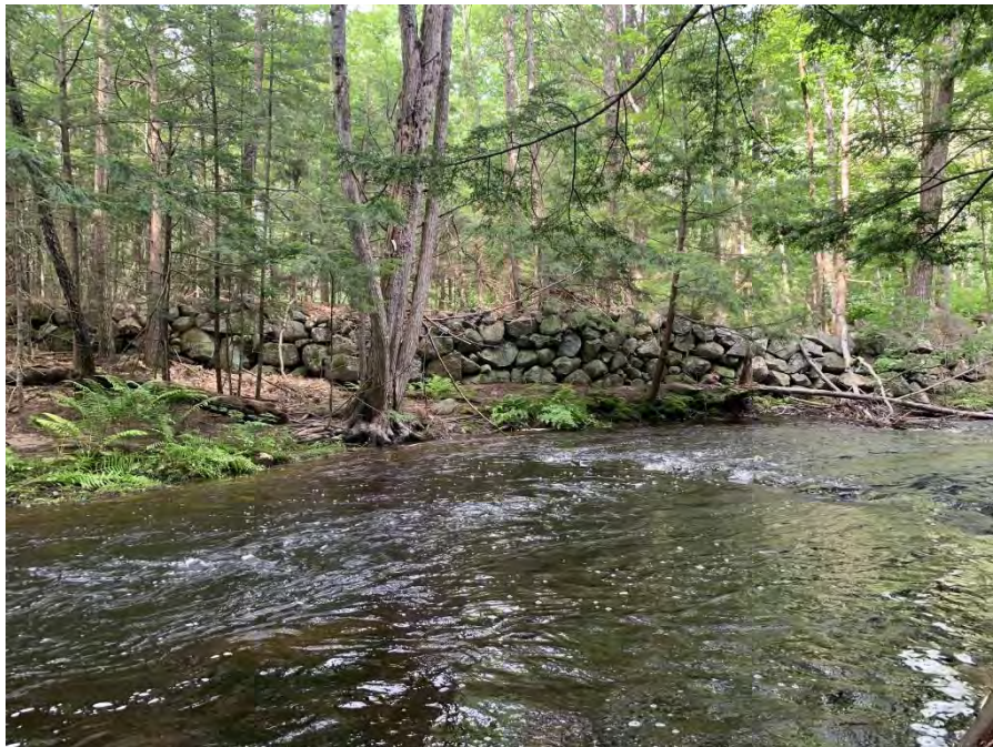
Photo 8. Dry-stacked boulder wall running parallel to the river upstream of the High Street Crossing.
