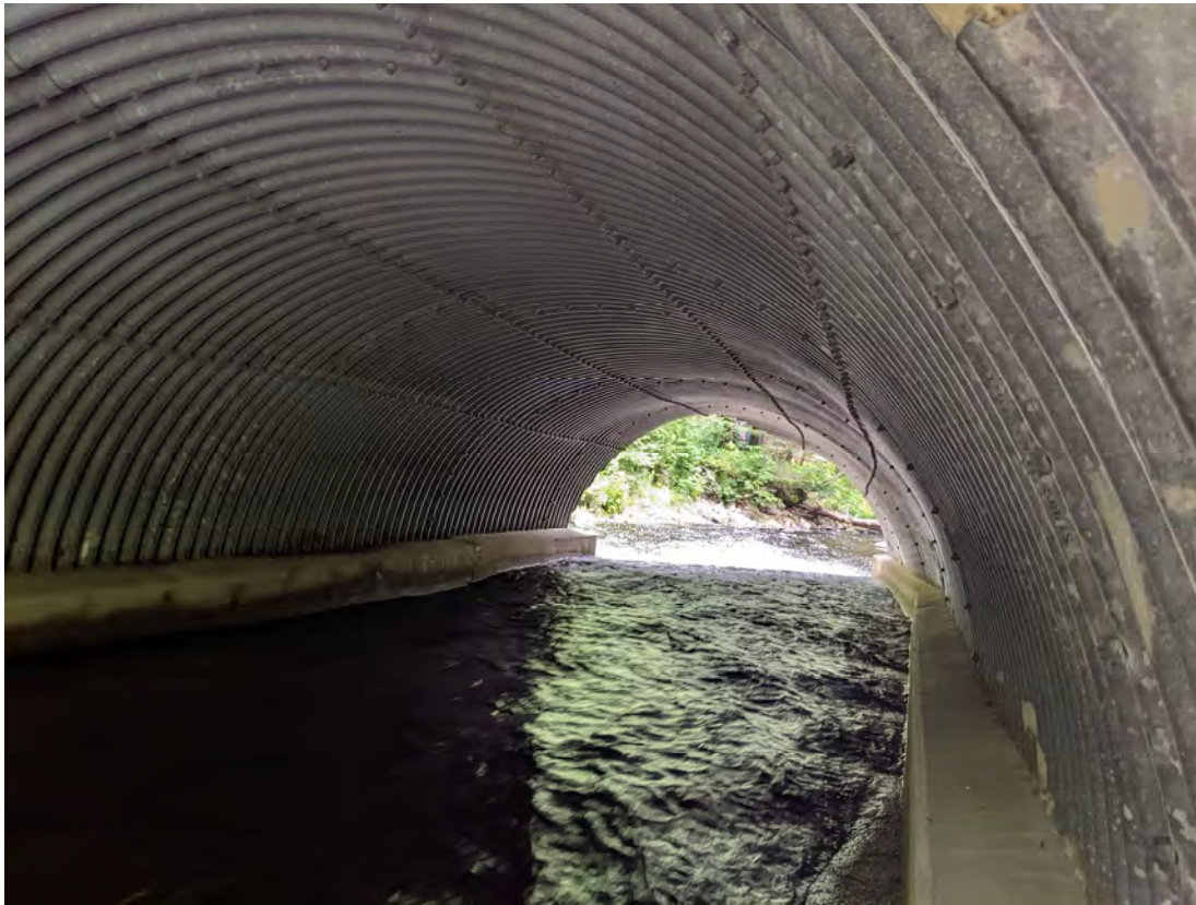
Photograph 25: Culvert conveying Melvin River beneath High Street
