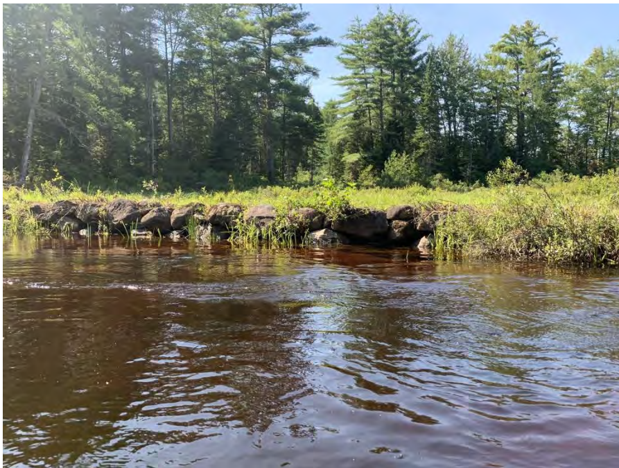
Photo 20. Newly cleared riverbank and boulder revetment along Reach 2b.
