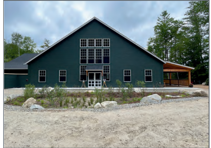
Retention Basin to collect and filter runoff
