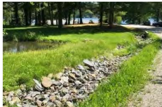
Rock-lined swale (Source: VT Dept of Environmental Conservation)
