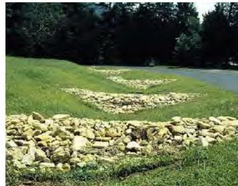
Grass swale with stone check dams (Source: LakeSuperiorStreams.org)
