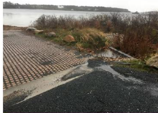
Boat ramp with concrete dip diverting runoff to bioretention (Credit: HW)
