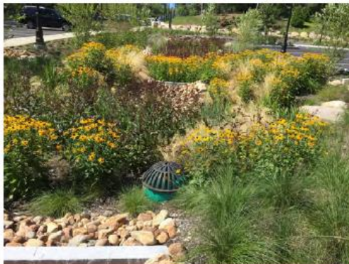
Bioretention basin (Credit: HW)
