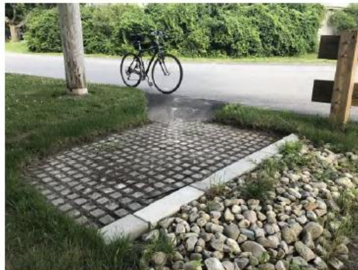
Sediment forebay with paver mat and level spreader (Credit: HW)
