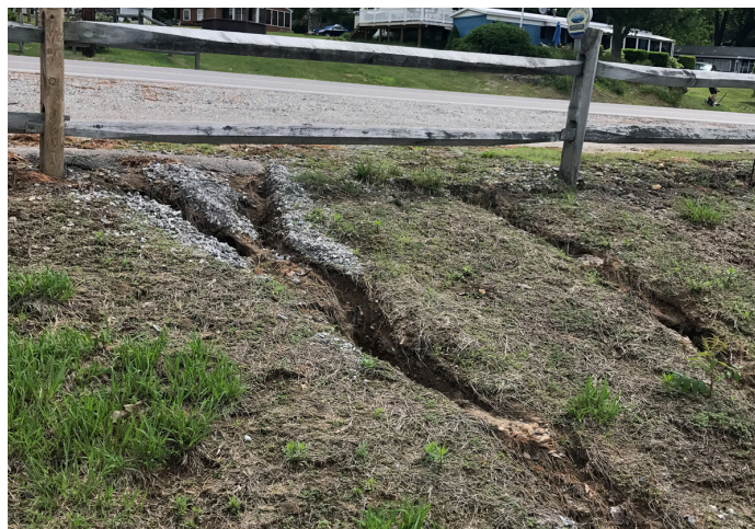
Erosion present from stormwater on Weirs Blvd. to Langley Cove.
