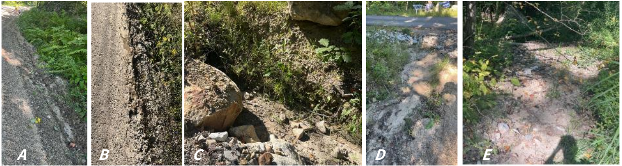
(A, B) Road shoulder gullies lead toward a wetland. (C) View of a stormwater culvert on Jesus Valley Road. (D) Outwashed sediment on the road shoulder suggests that stormwater carries pollutants downslope. (E) Sediment from the road deposits into the forested area.
