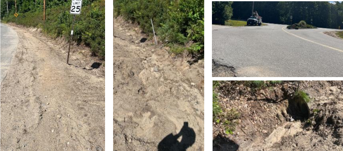
(Left) The road ditch is on Route 11-D is completely bare. (Middle) Multiple small gullies run through the ditch. (Top right) Large impervious area at the intersection of Route 11-D and Mount Major Highway. (Bottom right) Stormwater exits the ditch through a culvert.
