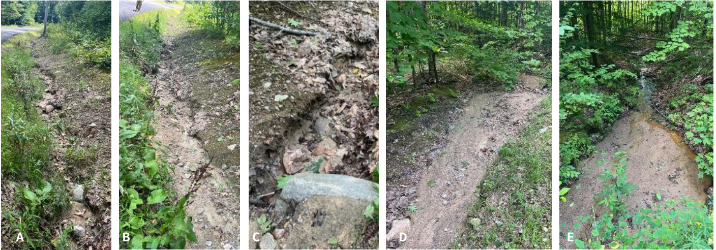
A, B, & C: The large gully on Alton Mountain Road leads directly to a stream. D & E: Sediment has accumulated at the intersection of the road ditch and the stream channel.
