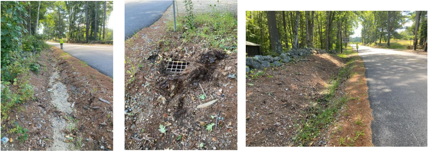
(Left & Right) Photos of the ditch showing accumulated sediment. (Middle) Accumulated debris around the catch basin.
