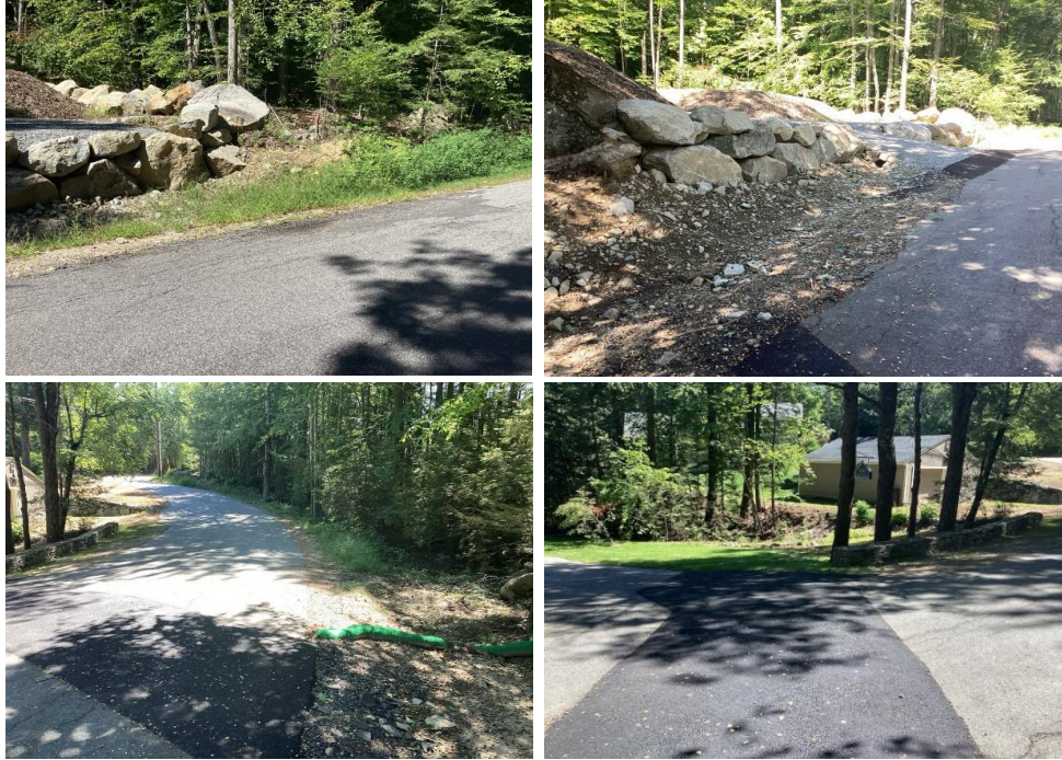
(Top Left) Sediment is washing out from the construction site onto the road shoulder. (Top Right) The unvegetated ditch downslope of the construction site is eroding. (Bottom Left) An existing filter sock in the ditch is overtopped by sediment. (Bottom Right) A view from Echo Shores Road, looking north towards the culvert outlet next to House 122.
